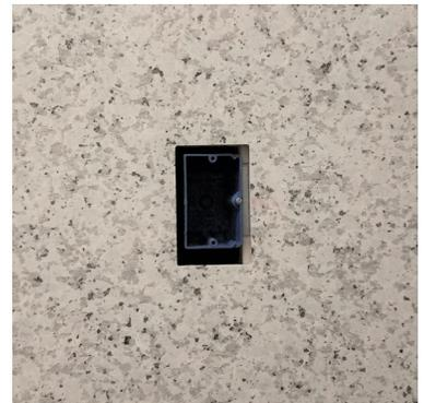
3. Insert the Smoothline wall flange. Glue the flange to the stone using a glue that is compatible with the solid surface. It may be easier to glue the flange in before installing the stone.
